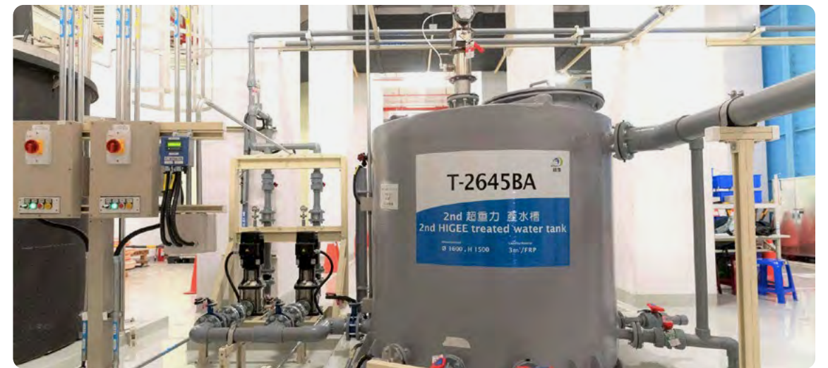
TSMC extends the application of high-gravity rotating packed bed technology to ammonia nitrogen wastewater treatment.
