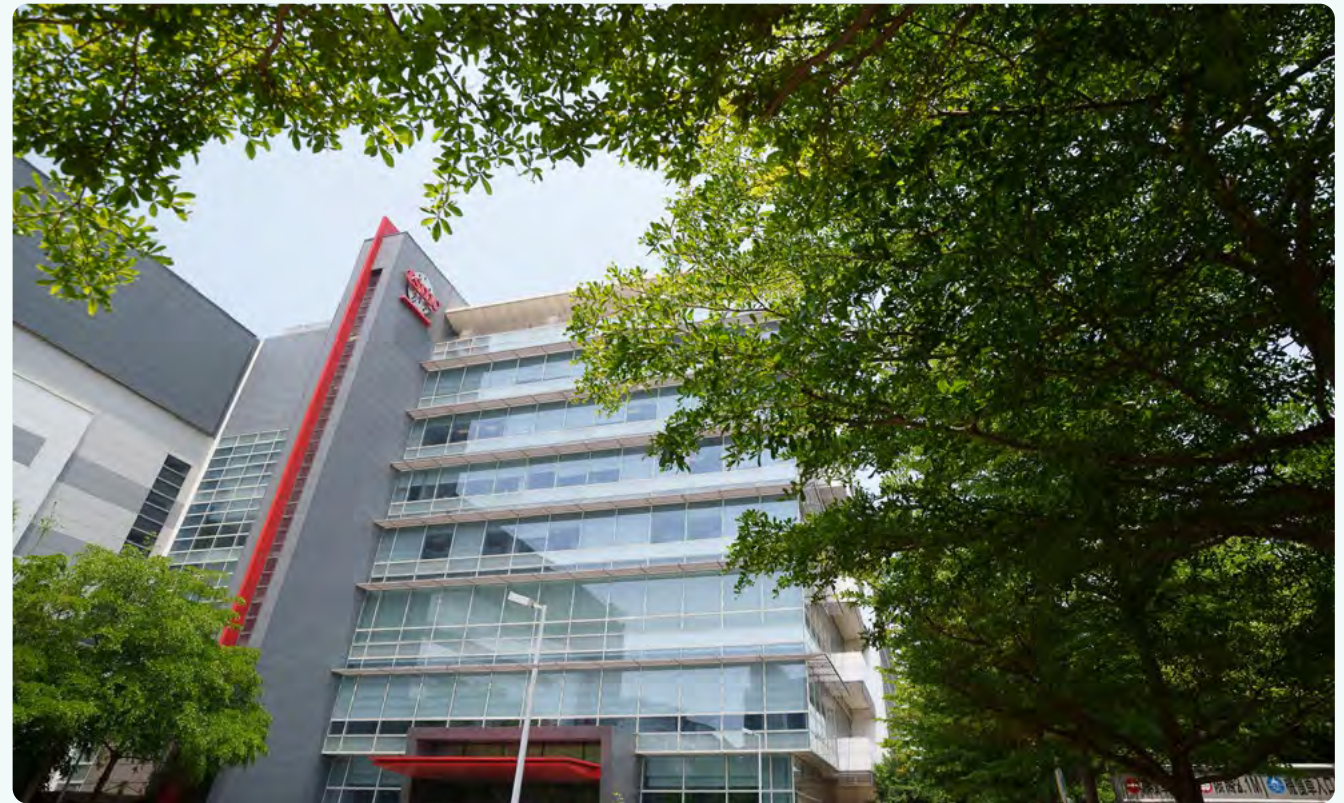
TSMC introduces reclaimed water into fabs with advanced processes.
